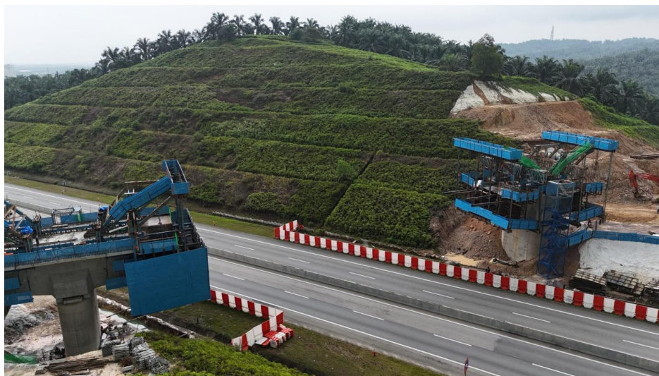
Fig. 1: The site condition for Bridge 18 crossing LATAR Expressway
