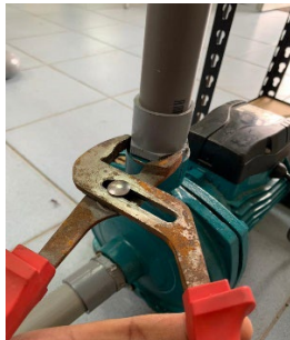
Figure 11: Installing the pump
