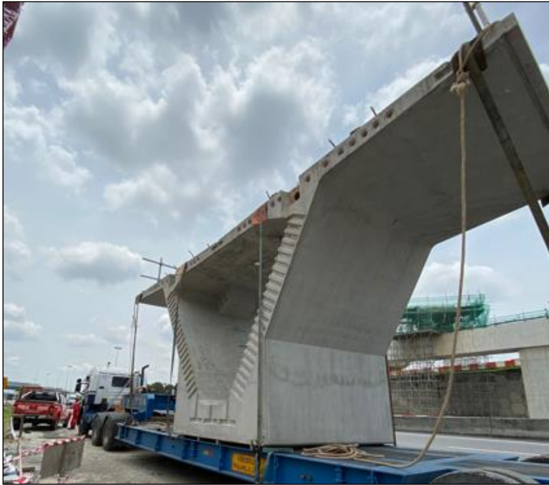
Figure 1: Segmental Box Girder (SBG) at LRT3 Construction Site
