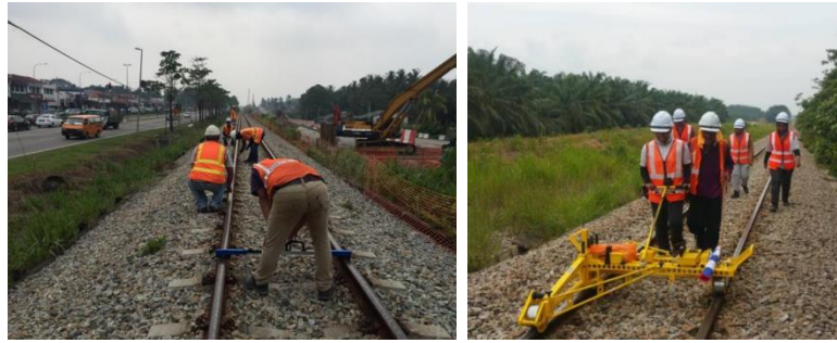
Figure 2: Manual Gauge activity and Running KRAB 84.09 activity
