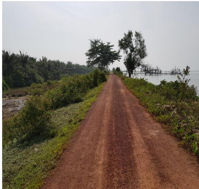
**Figure 1: Overlying service road of coastal embankment in Senggarang Batu Pahat**
