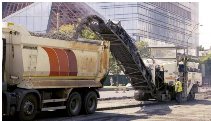
Figure 2: Asphalt milling machine
