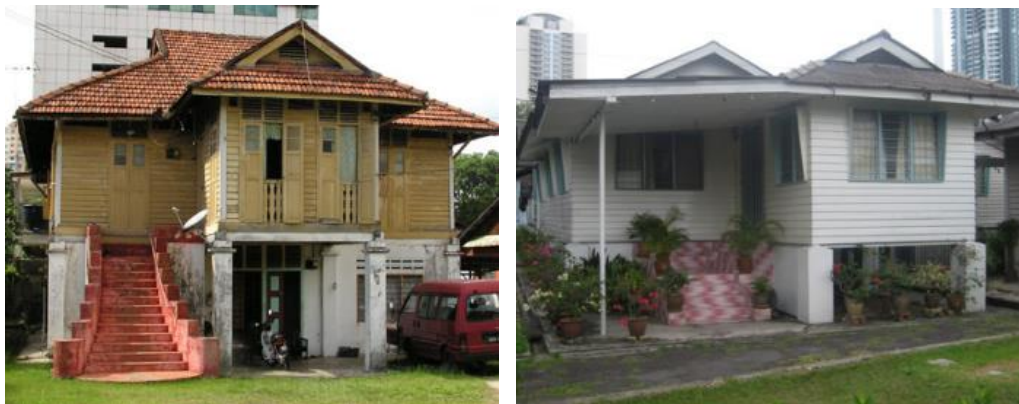
Fig 1 Modernized Timber House (source: Ju et al. , 2012)
