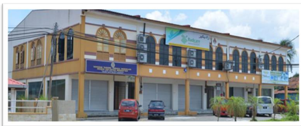
Figure 3: Building at Jalan Dato Lundang Business Building, Kota Bharu.
