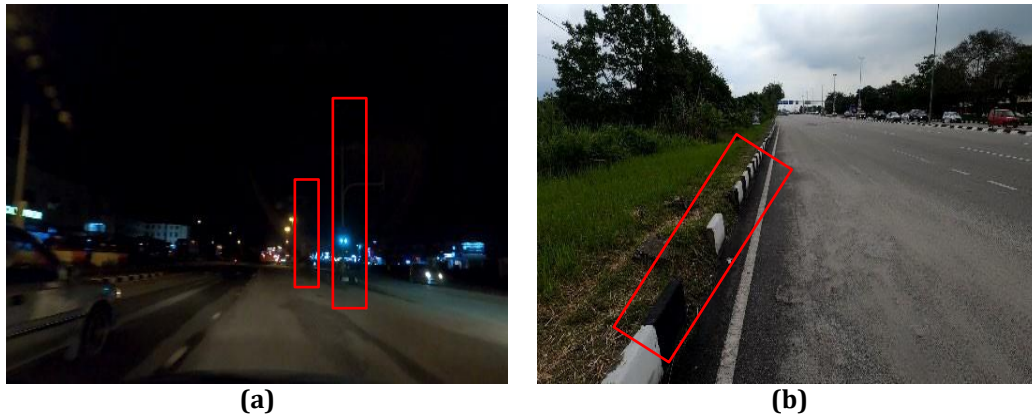
Fig. 6 Road Furniture Condition (a) Malfunction Streetlight; (b) Missing Kerbs
