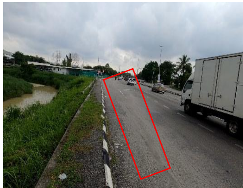
Fig. 7 Faded Road Making
