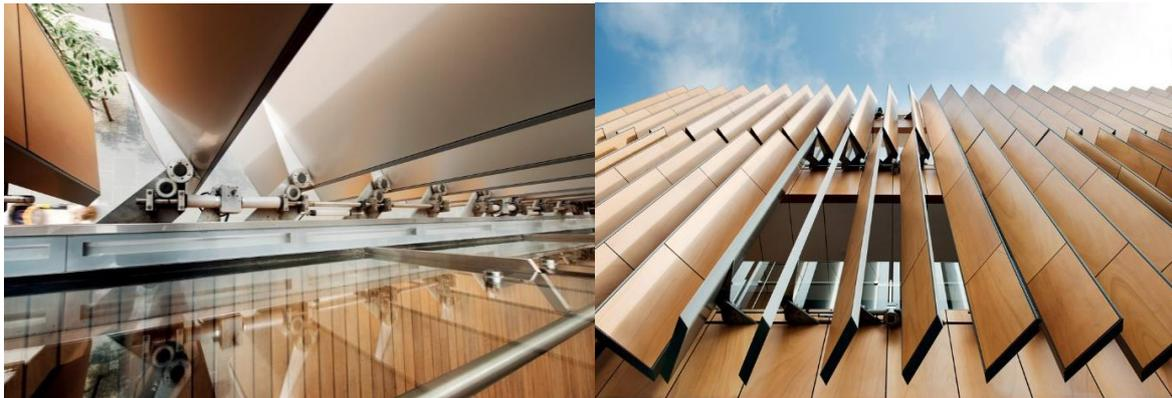
**Figure 4: The shading devices louvres [7]**
