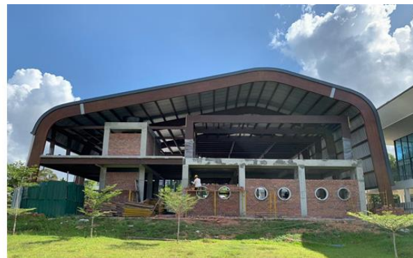
Figure 2: Rear view of engineered timber building in Johor Bahru
