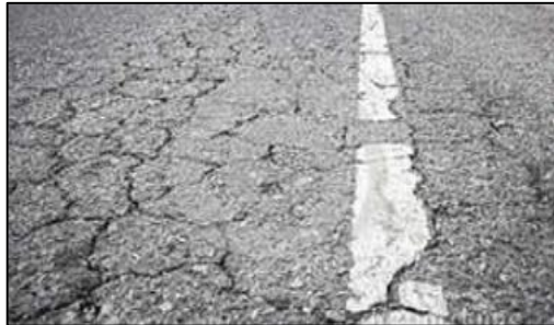
Figure 1: Deformation of fatigue cracking [15]
