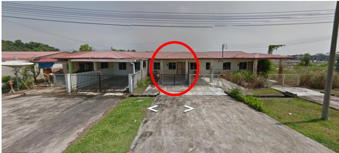
Figure 1: Location of the Terrace Urban House
