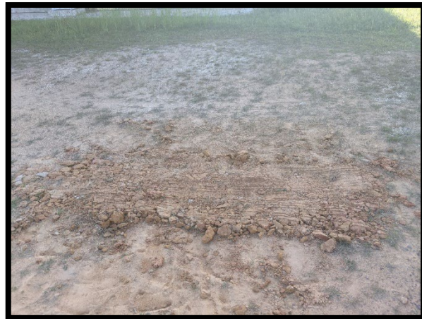
Figure 11: Test Area 2 after compaction
