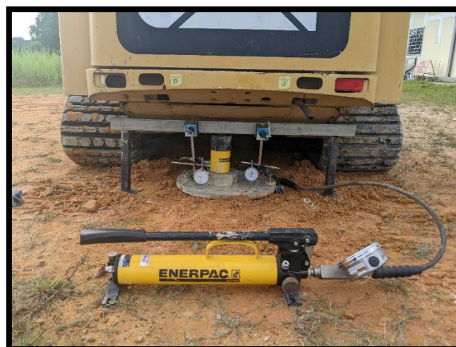
Figure 12: Plate bearing test setup at Test Area 2
