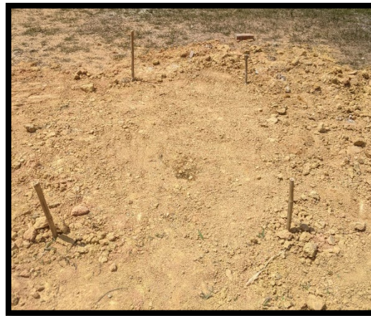
Figure 9: Test area 1 after compaction
