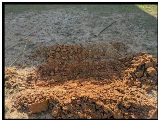
Figure 10: Excavation of soil
