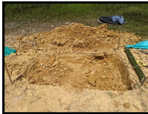
Figure 7: Excavation of soil
