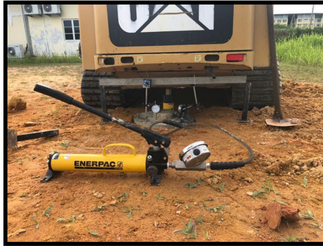
Figure 13: Plate bearing test setup at Test Area 1
